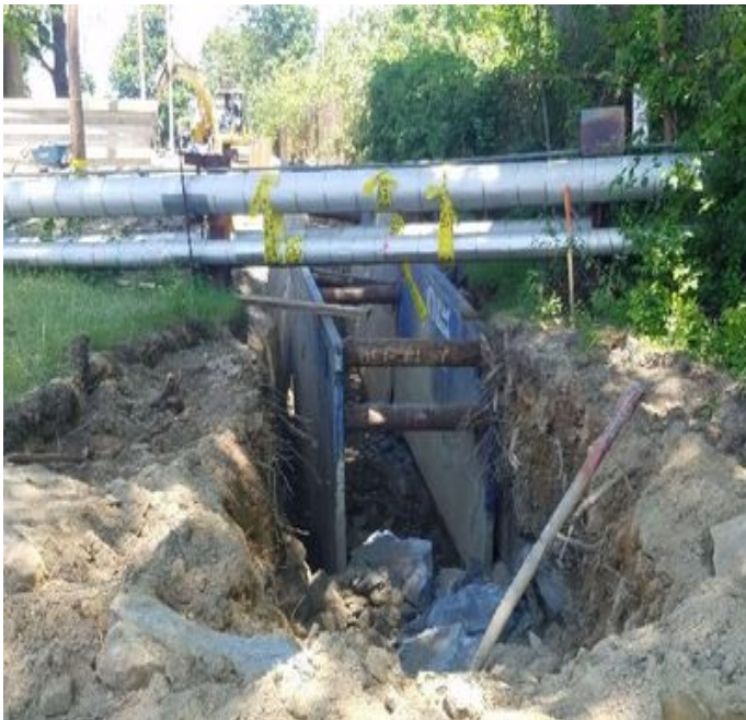
Fig 11: Excavation next to the field house, under steam pipe. Viewing north. (6-24-19).
