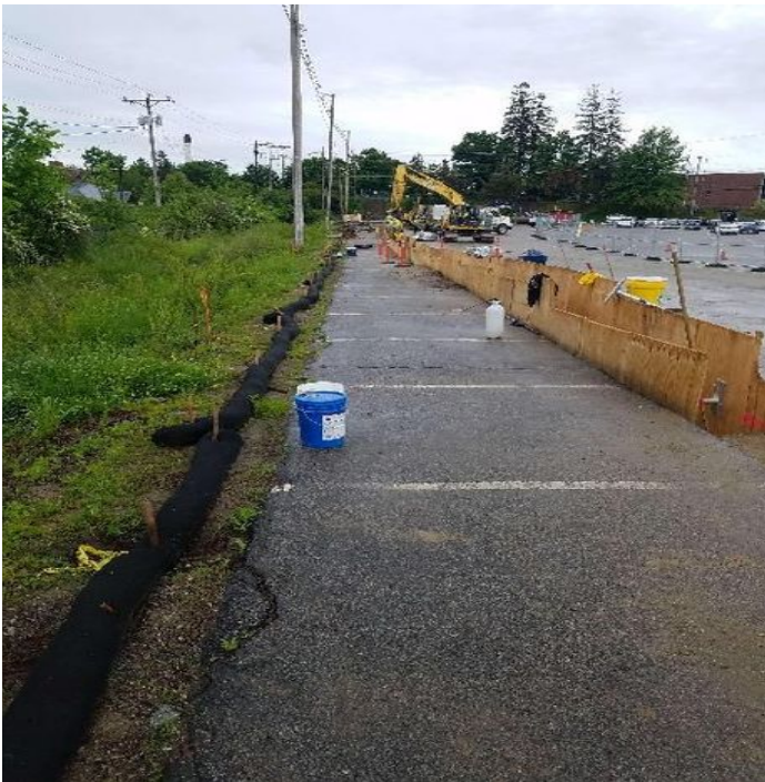
Fig 3: Silt sock installed along trenching activities in "A" lot. Viewing south. (6-21-19).
