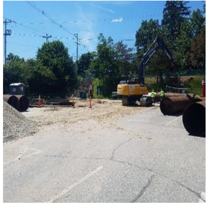
Fig 10: Midwest Mole Inc. Prepping to begin drilling this week. Viewing south. (6-24-19).
