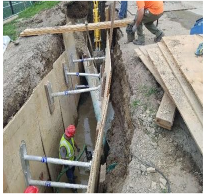
Fig 18: McCourt pumping water out of trench into existing trench. Viewing north. (6-25-19).
