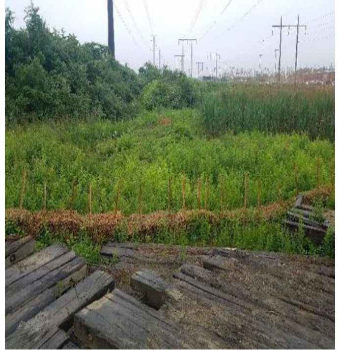
Fig 22: Straw bales installed between Str. F107-138 and wetland NW37. Viewing west. (6-25-19).
