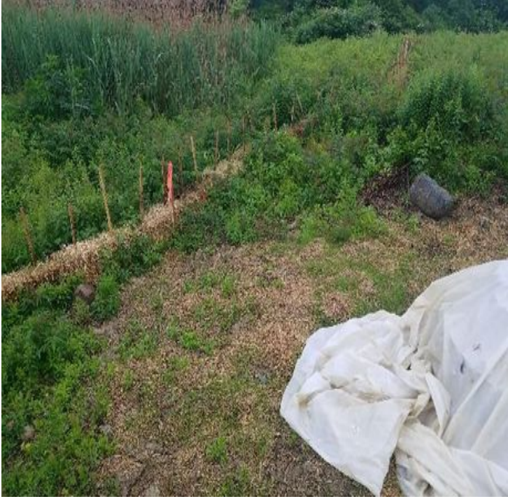
Fig 21: Straw bales installed between Str. F107-138 and wetland NW37. Viewing north. (6-25-19).
