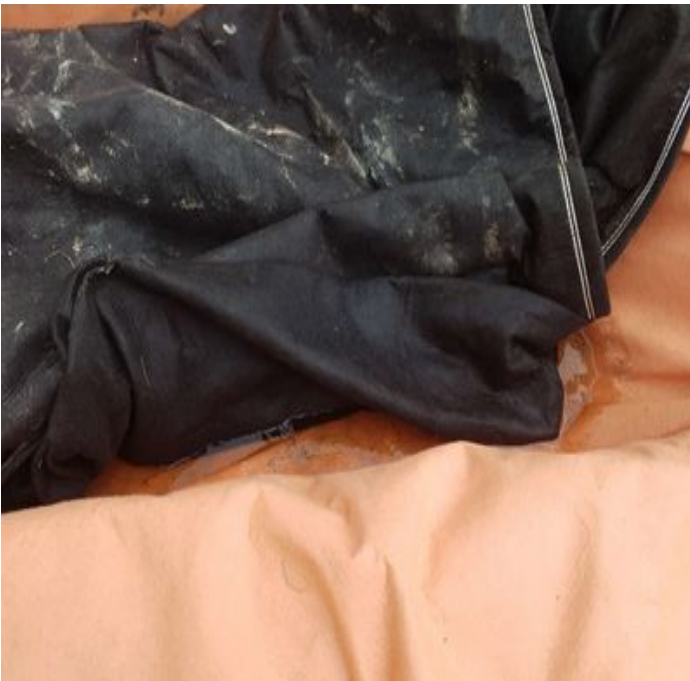
Fig 7: Rain water filtering out through the filter bag inside the dewatering Apparatus. (6-21-19).
