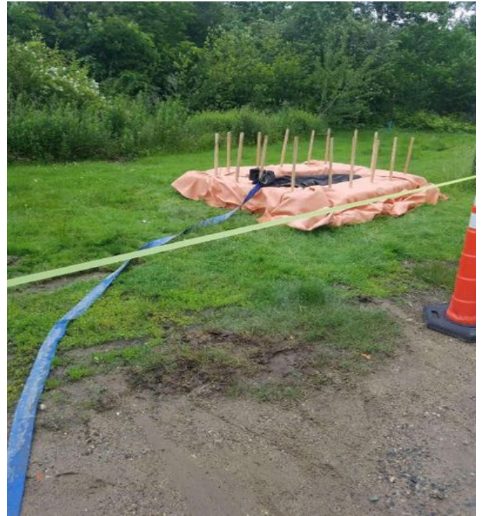
Fig 6: Rain water pumped across Colovos Rd into dewatering apparatus. Viewing southeast. (6-21-19)
