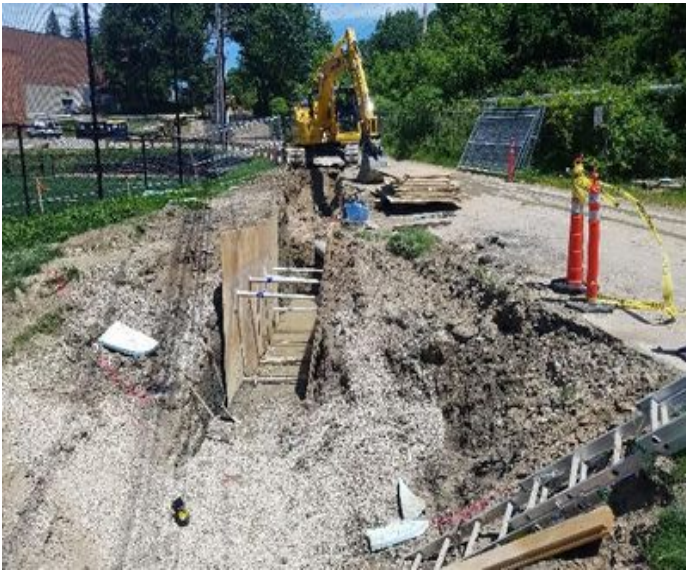
Fig 13: Excavation north of trench along Colovos Rd, moving towards steam pipe. Viewing north. (6-24-19).
